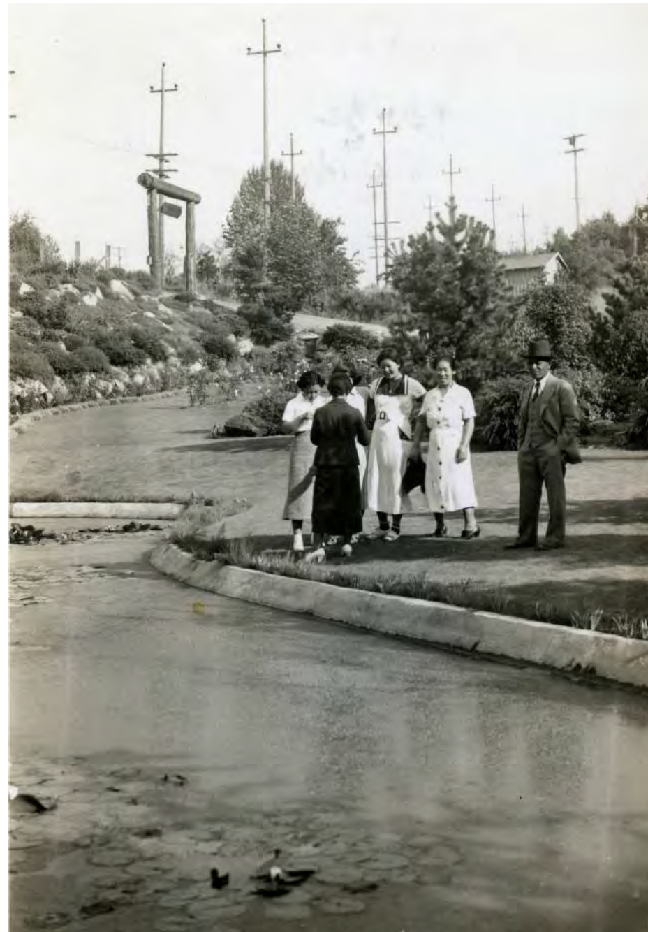
Lily Pond with the Rockery Wall Showcase and Entry Gate in background Source: KGF Photo #1983, dated 1935
