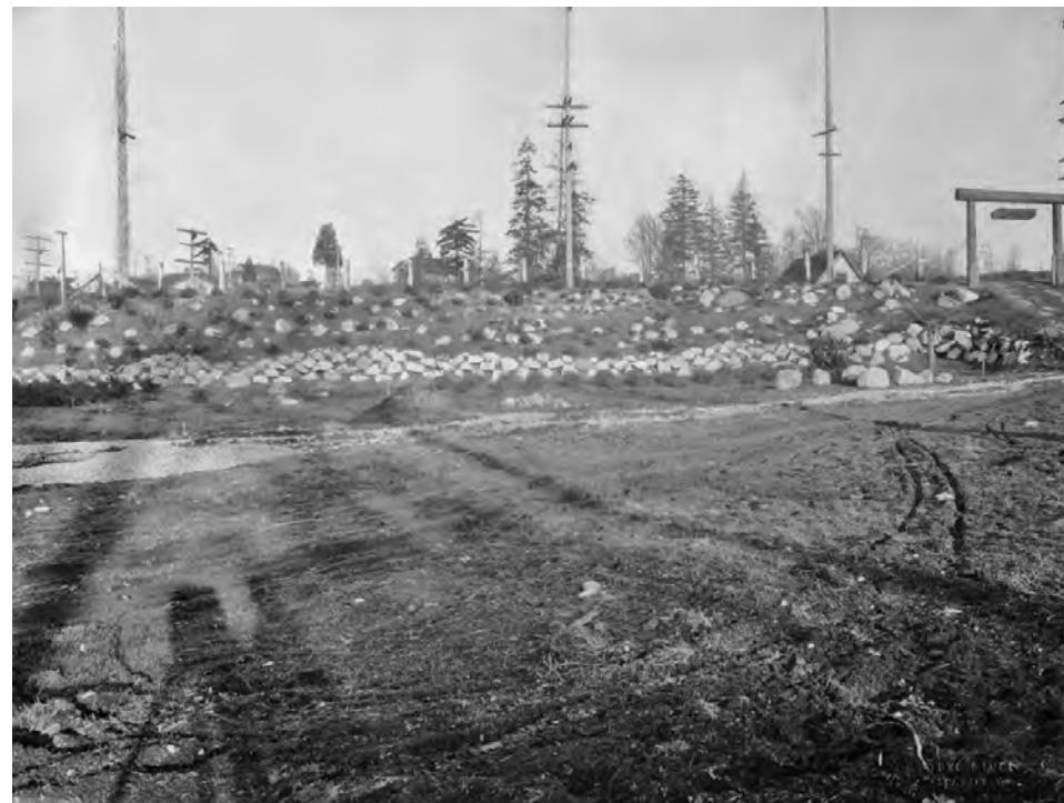
Looking north, view of the Rockery Wall Showcase with Renton Avenue above, log entry gate on the far right. KGF Photo #46, dated 1930.
